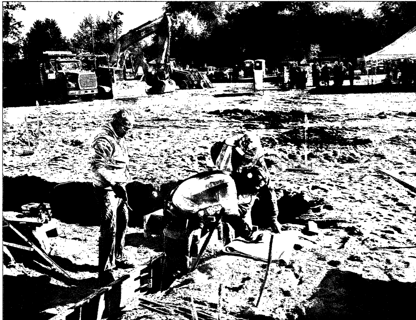
Mike Napier, Mike Napier Jr. and James Dean of J.C. Holly Construction work at the site near the the groundbreaking for the Farmers Market pavilion and other improvements to Tattan and Central City parks. PHOTOS BY BILL BRESLER | STAFF PHOTOGRAPHER
