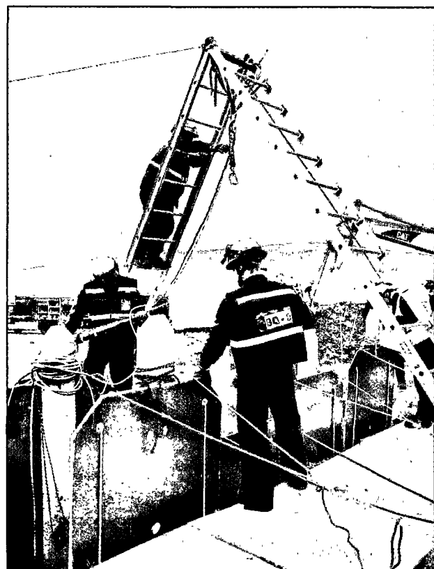
Stabilizing the trench walls and building the tower that supports the Vactor hose.
