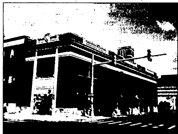
A former Detroit firehouse has been transformed into the University of Detroit Mercy's George J. Asher Law Clinic Center.
