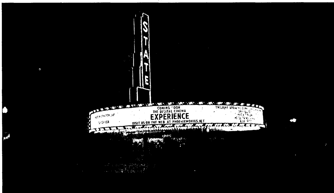
More than 530 lights and the electronics have been restored on the State Wayne Theater's wrap-around marquee. In all, there are 1,152 lamps, 550 which stay lit and 602 on a "chaser" to light up the downtown streetscape.
