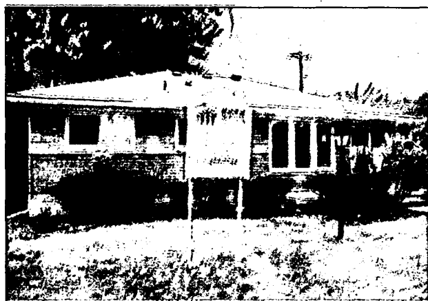
This renovated house on Julius is the latest Habitat for Humanity of Western Wayne project in Westland.
