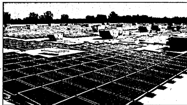
IKEA this week officially plugged in the solar energy system installed at its Detroit-area store in Canton, the state's largest such photovoltaic array.
