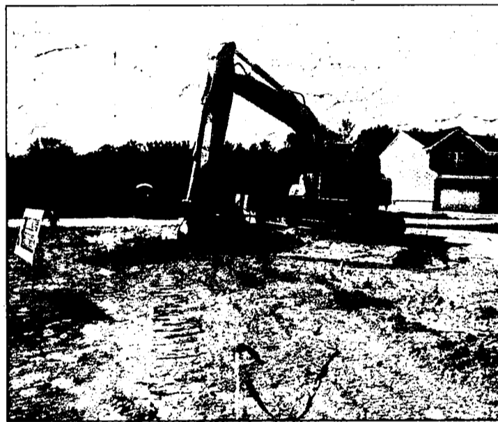
Builder Rick Elkow officially breaks ground to begin construction for the first home in the Made in America/Built in Michigan initiative in Howell.
