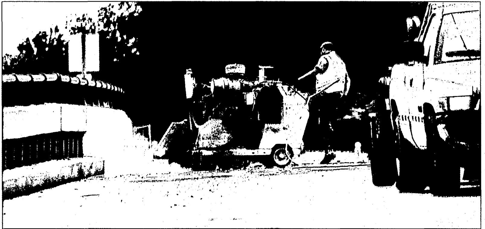
Work on the Warren Road bridge over I-275, already under way, is expected to last through September.
