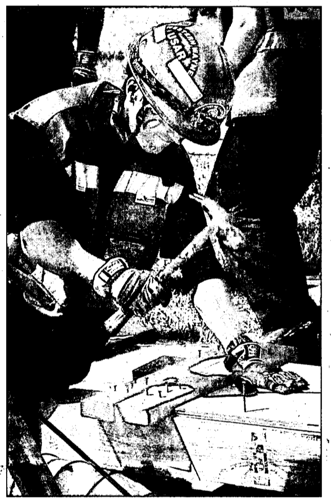
One of the first jobs is to build a bridge to enable rescue workers to work directly over the trench.
