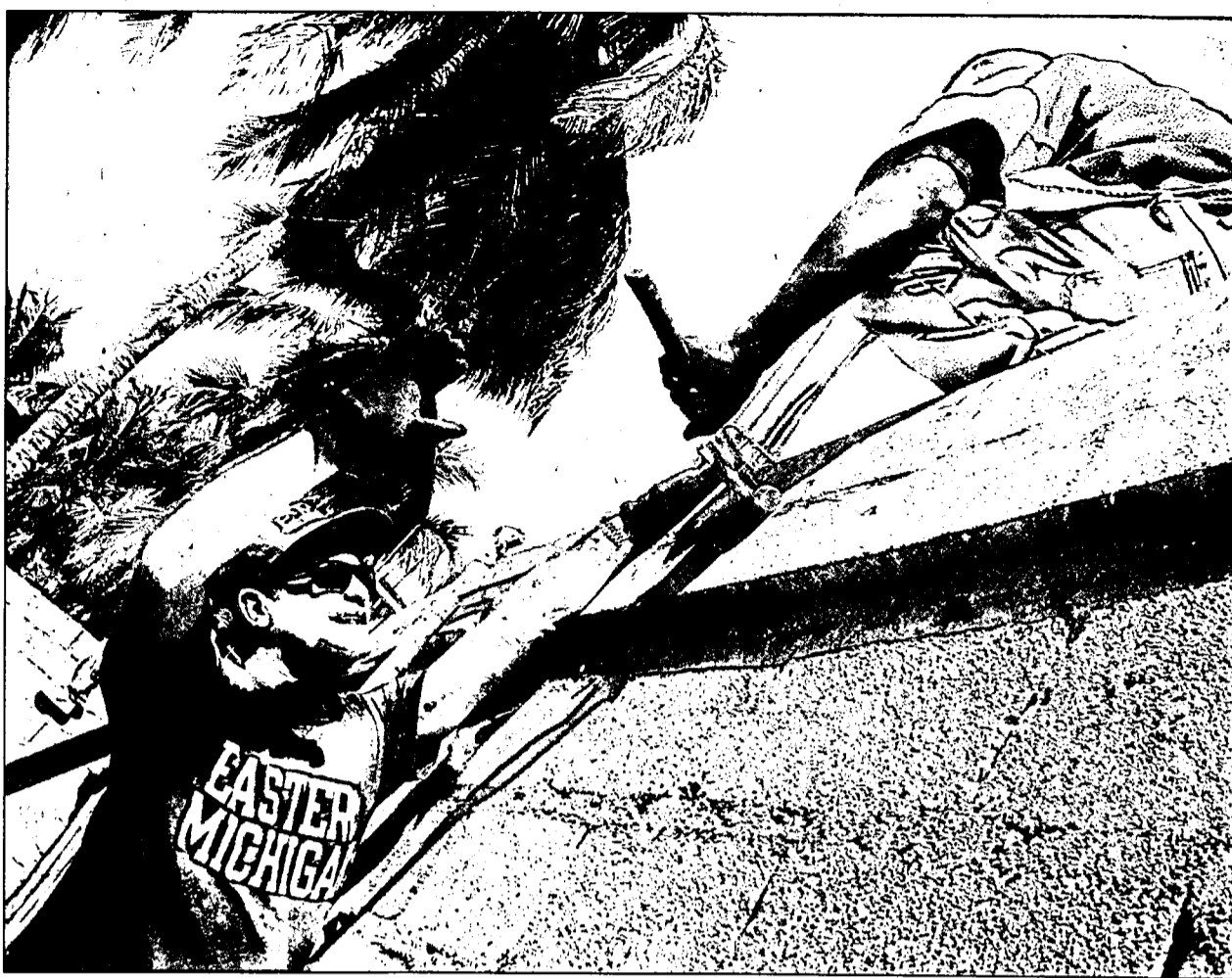
Paul DeNapoli of Livonia works on a safety wall in Haiti.
