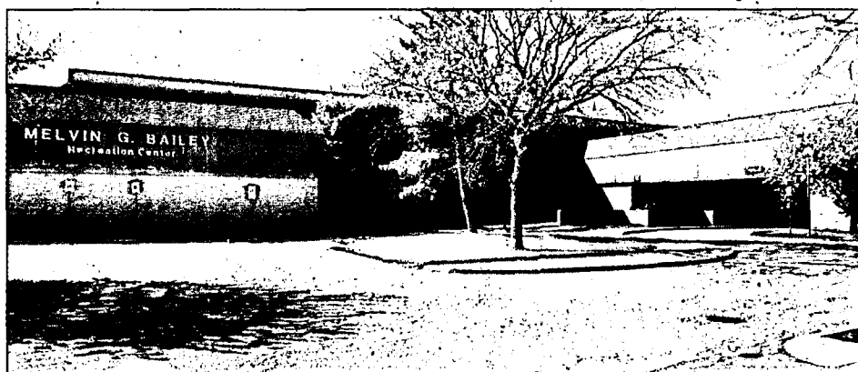
Built in the late 1970s, The Bailey Recreation Center and its outdoor pool are slated to close for good at the end of June and recreational services taken over by the City of Wayne.
