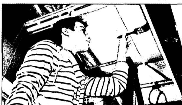
Patrick Tirney paints the soffit of the shed white. They will be covered in vinyl siding provided by Siding World.
