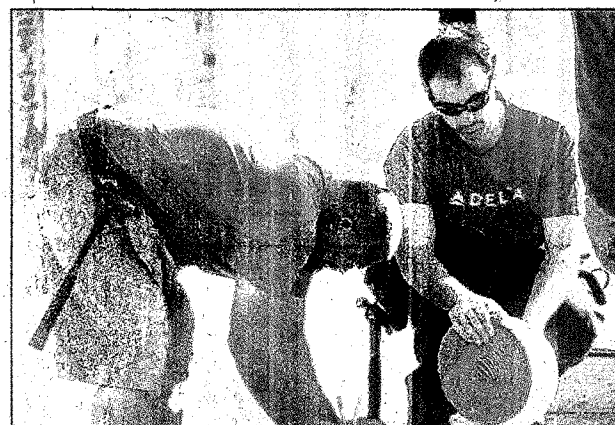
Delta employees Greg Bursvold and Jason Bucceri work on the home.
