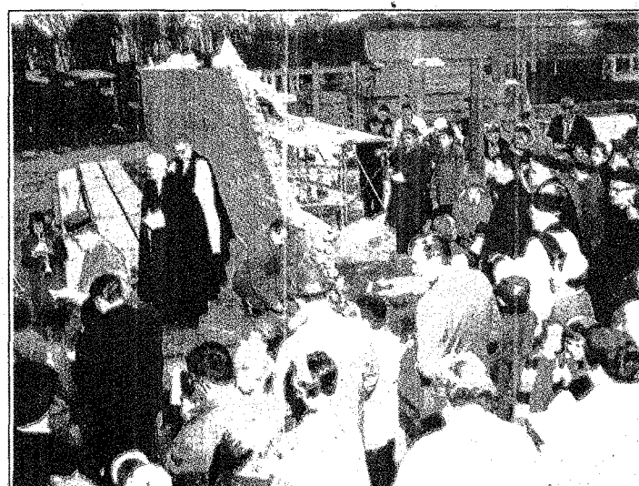
The congregation gathers to place the cornerstone of the church on Sheldon, Nov. 15, 1959.
