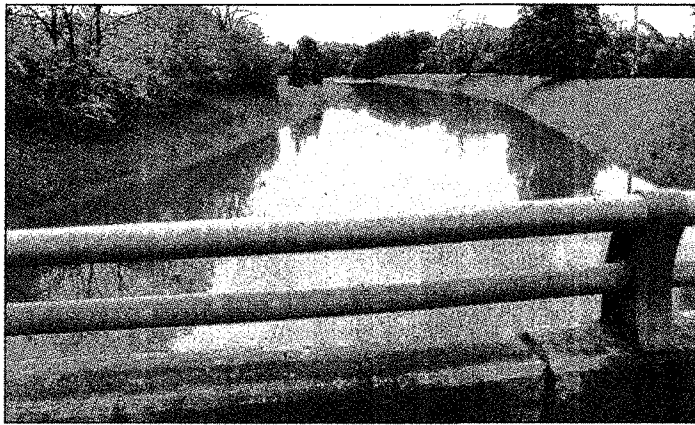
Hines Drive near Warren Road in Westland couldn't be seen under the Middle Rouge River which spilled over its banks after heavy rainfall Wednesday.
