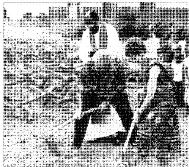
Paul and Nancy Berrigan of Farmington Hills dig their shovels into the ground in Chelekura, a remote area in Uganda, where a new science and library building will be added to the campus of their John Paul School.
