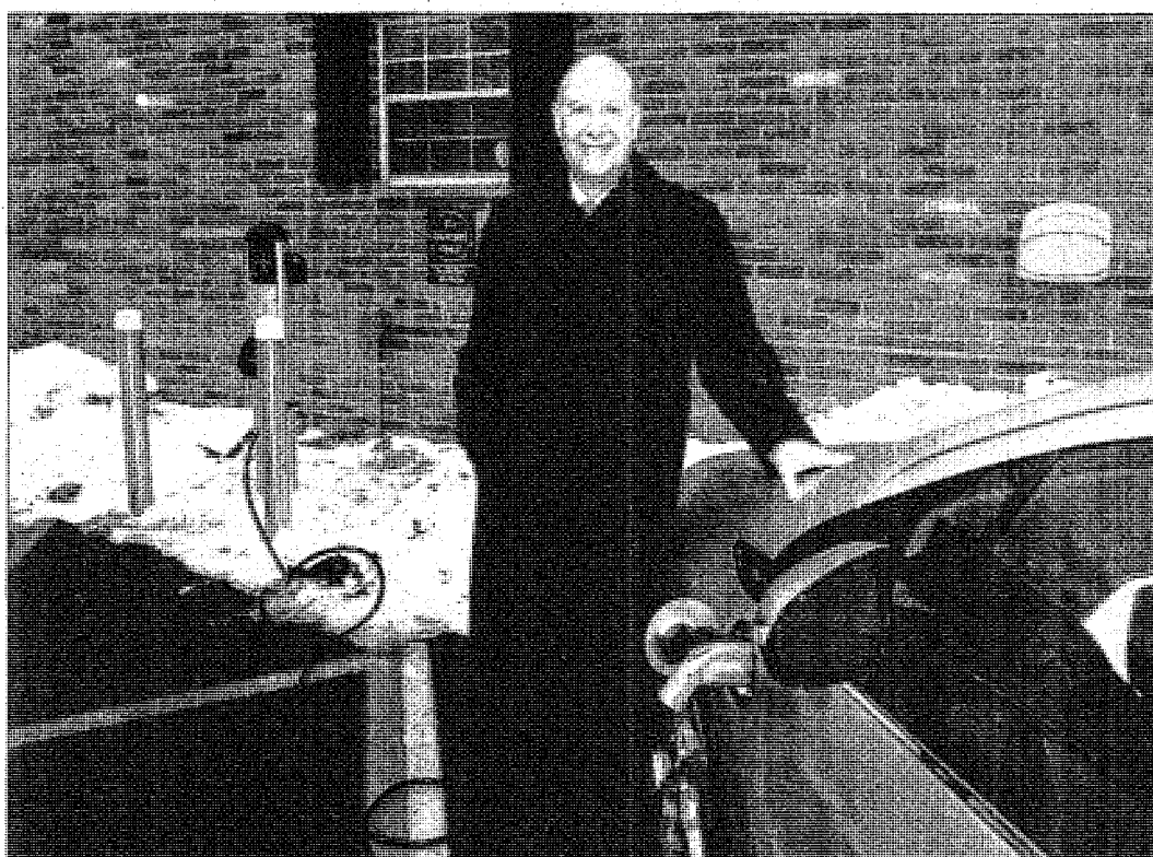
Westland Colonial Village Apartments owner Jeffrey Spoon poses with a Chevy Volt plugged into the new electric charging station - the only one installed at an apartment complex in the country.
