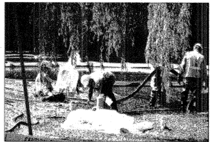
Booms along Talmadge Creek in Calhoun County steer the oil to the shore where workers wearing respirators are vacuuming it up.
