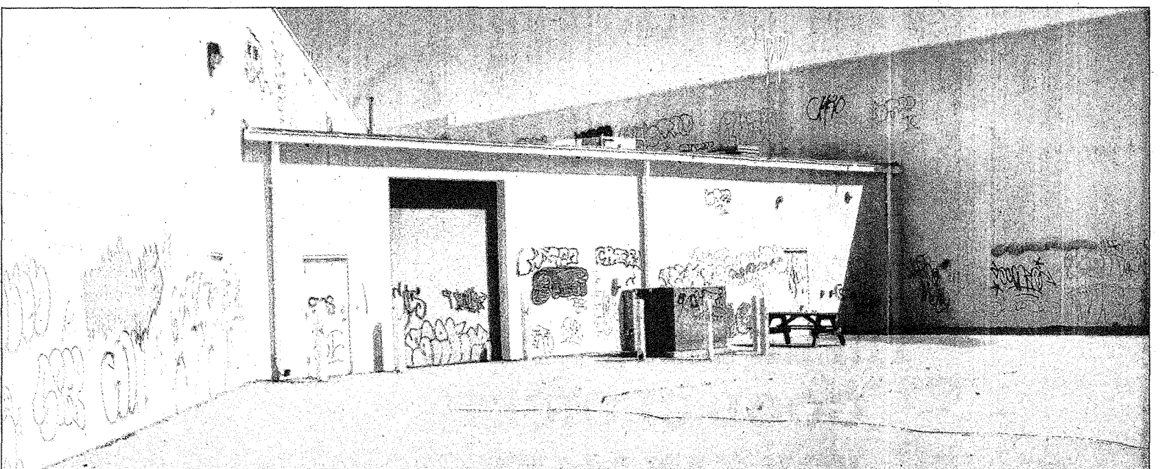
Three men have pleaded guilty to spray painting graffiti on three walls at the rear of the Value City building on Warren Road, in Westland. Cleanup is estimated at more than $14,000.
