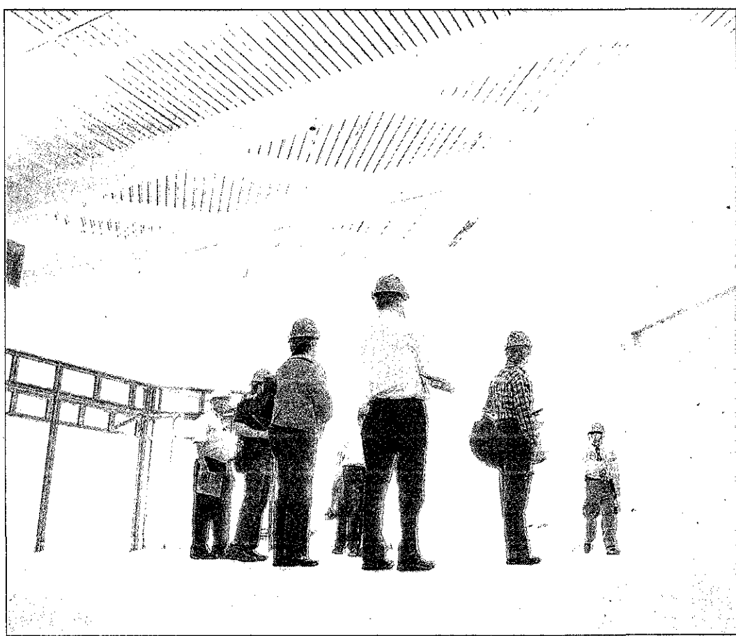
The new terminal's design isn't as flashy as the McNamara Terminal, but will be a major improvement over the aged Smith Terminal.
