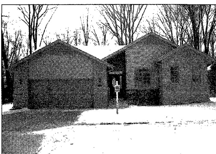
The Ashley, built by students in the construction technology program at the William D. Ford Career Technical Center is one of 62 homes featured in the 2008 Spring Parade of Homes.
