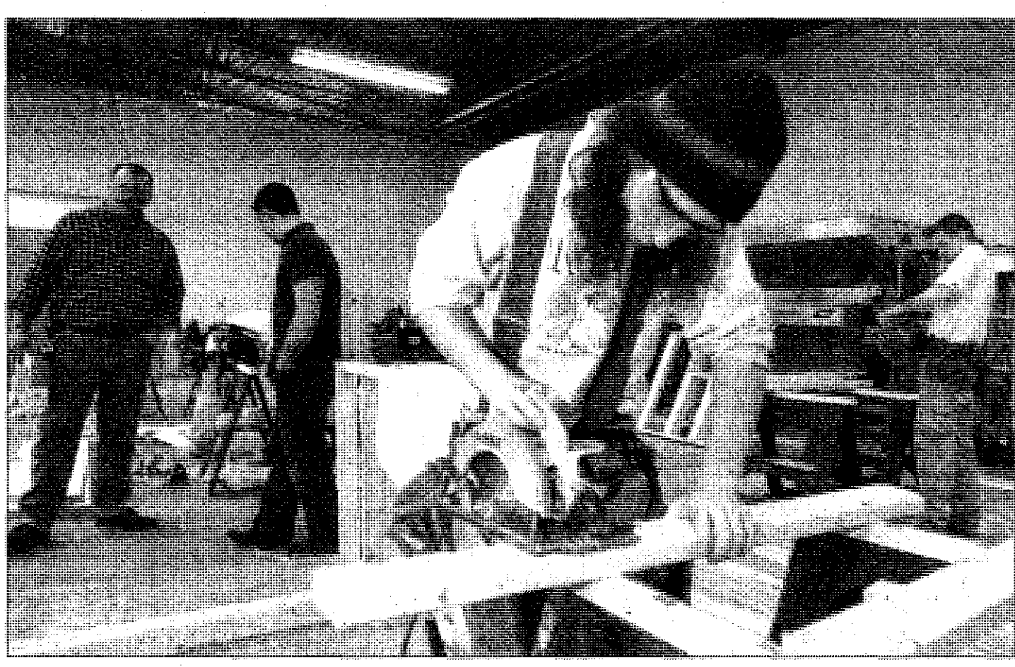
David Barber saws lumber for his structure as part of the SkillsUSA competition.
