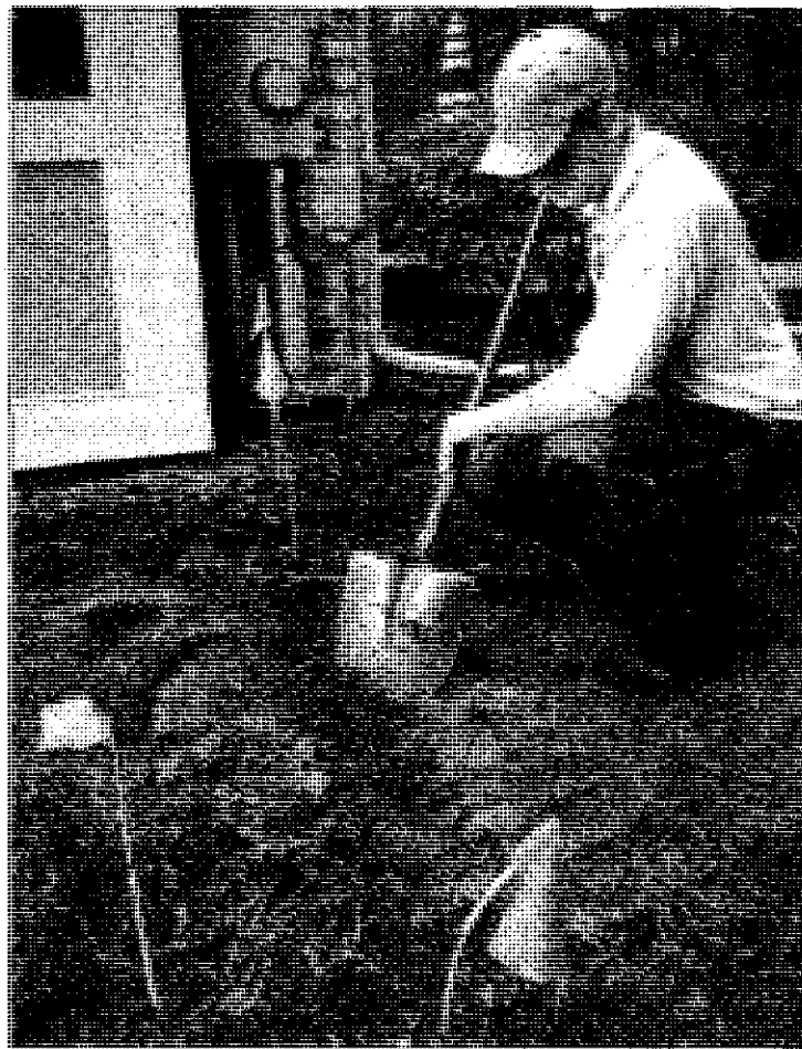
Professional landscaper Cliff Both, owner of Authentic Lawn & Tree in Cedar, Michigan, had a close encounter with a buried gas line early in his career that convinced him of the dangers of unsafe digging. He now calls MISS DIG to request staking before starting any job.
