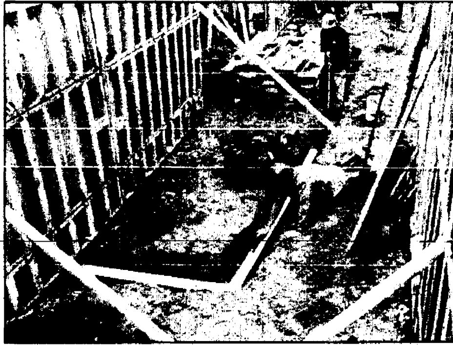
Building: Above, adult education student Brian Charlevois passes out a bucket of dirt at the construction site on Avondale in Westland. The home construction students are working on the conduit for the storm sewers. Below, students are making sure that the conduit is level for the storm sewer piping.
