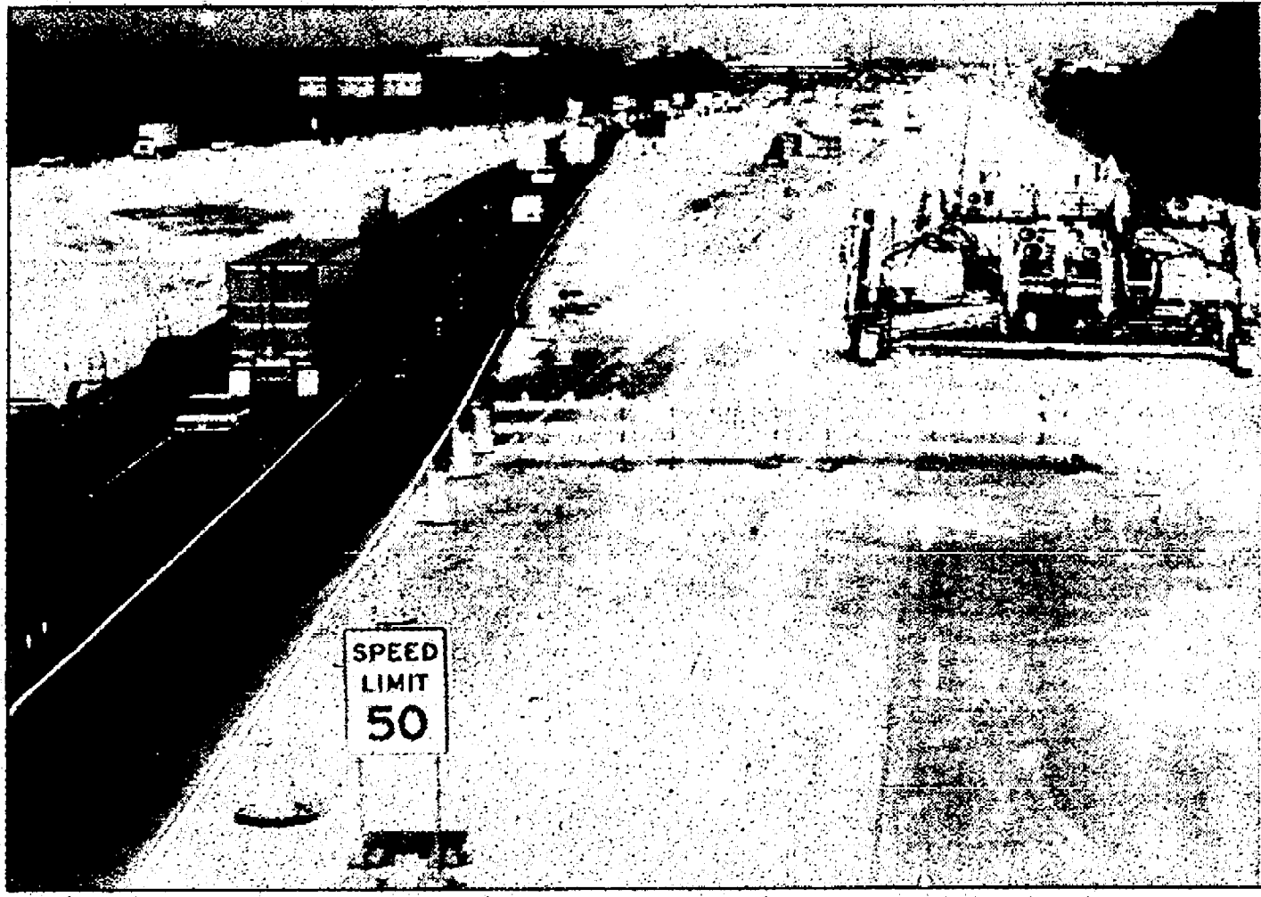
Intimidator: A spreader that can pour a concrete strip 36 feet wide was part of the equipment being used on the continuing I-275 paving project. This view is looking north from the Five Mile bridge.
