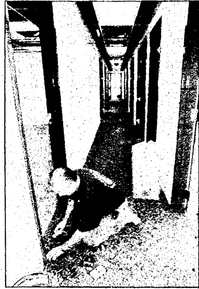
Hard at work: Tony Cerne of Quality Floor Co. lays new carpet at Adams Middle School. The target date approaches with Wednesday's start of school in the Wayne-Westland district.
