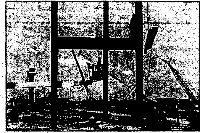
Girders rise: The steel frame is going up for the new mid-field terminal at Detroit Metro Airport.
