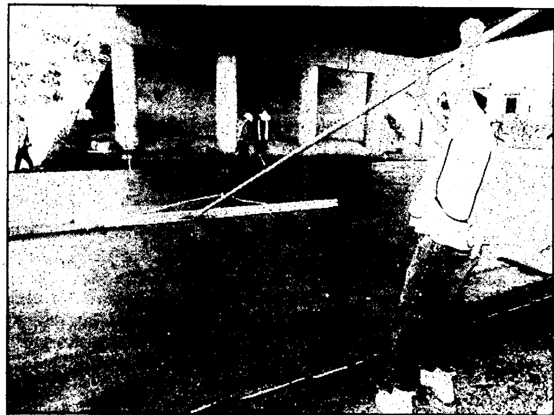
Mix'n' It up: One of two concrete spreaders shape and form concrete, above, for the new south-bound lanes of I-275. Road workers float the new pavement under the Grand River bridge.
