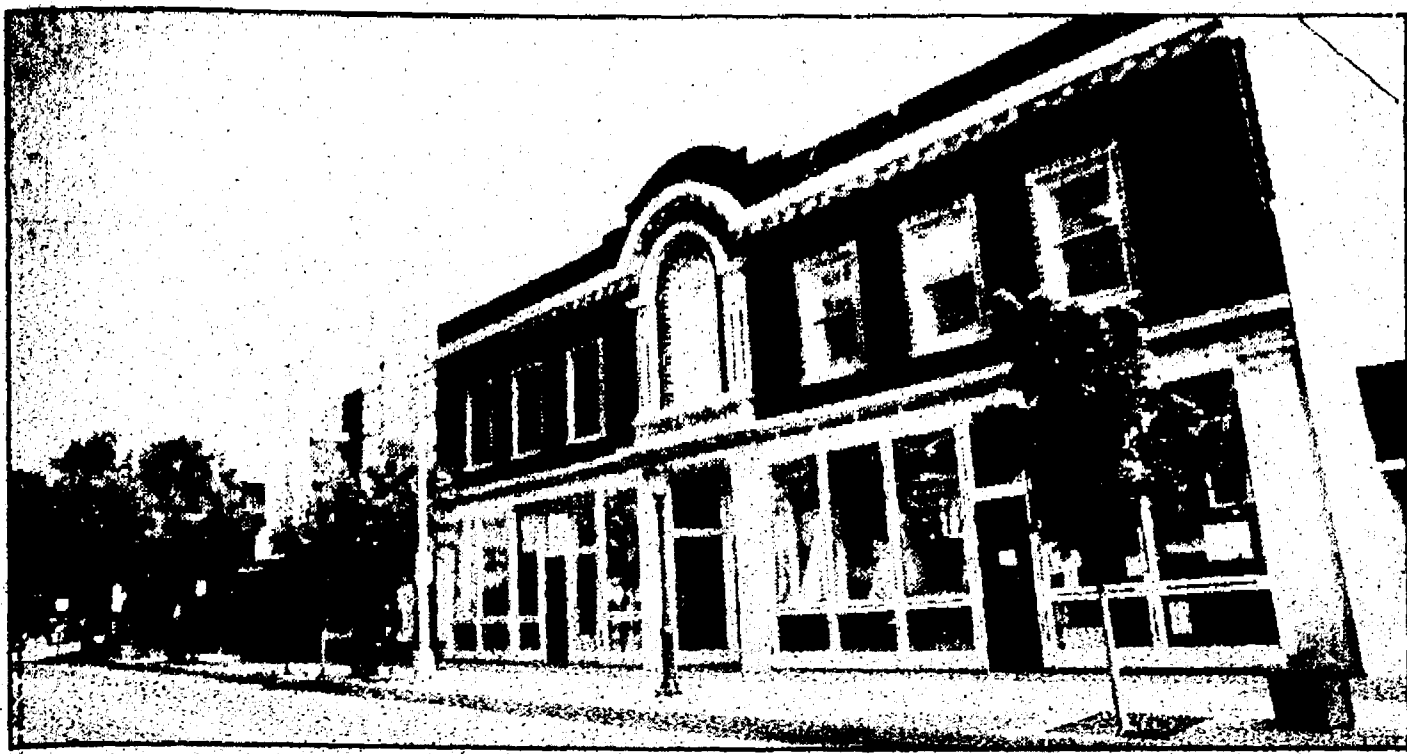
Downtown Farmington: New storefronts find homes in vintage buildings.
