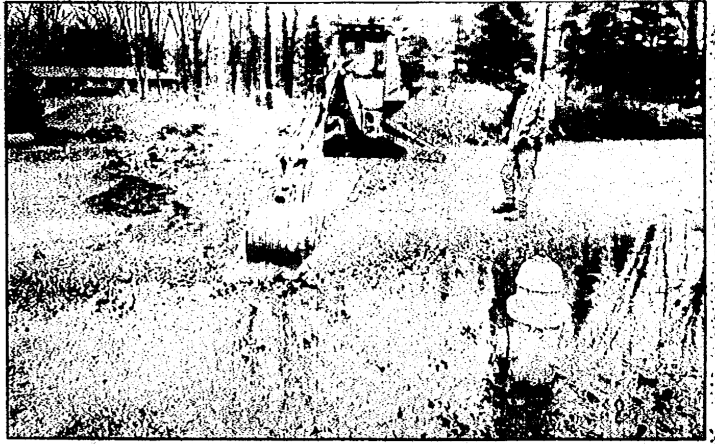
Dig It: City workers began digging a culvert on Tuesday in response to flooding on Ravine Street in Westland
