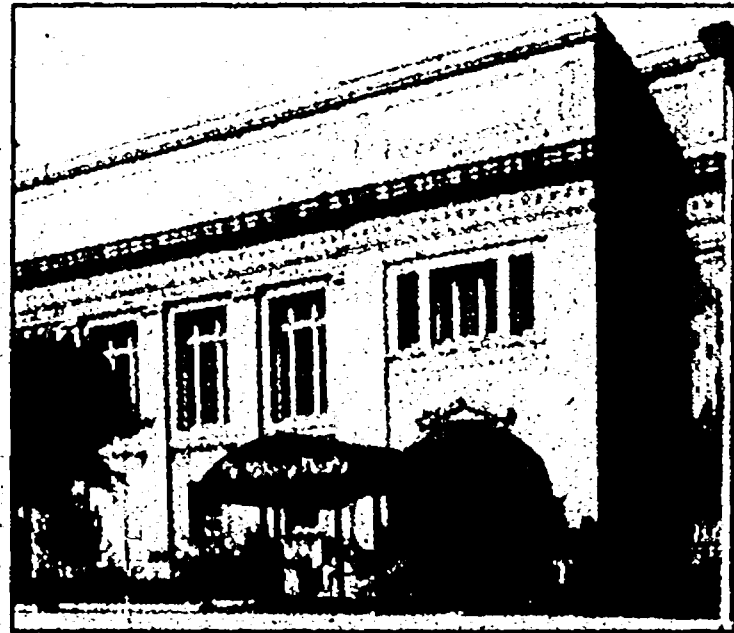
Well-known: The edifice of the Hilberry Theatre is as recognizable as its neighbor, Old Main, on the campus of Wayne State University in Detroit.
