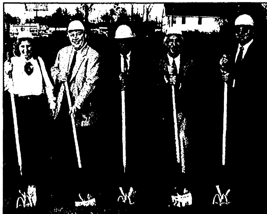
Dig It: The first digs of dirt to make way for a new prototype McDonald's in Westland were made by (from left) Dar Staley, manager of the new restaurant; Westland Mayor Robert Thomas; Norm Noble, construction engineer for McDonald's; Frank Martin, restaurant architect; and John O'Neil, operations consultant for McDonald's.
