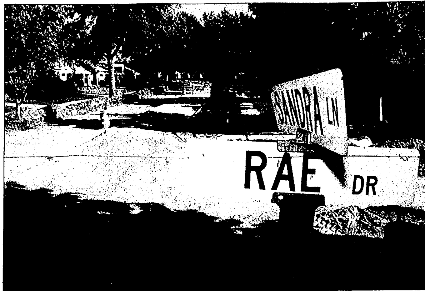
Under construction: A sewer-separation and street-reconstruction project has neighbors waiting for work to end in area bounded by Hubbard, Ann Arbor Trail, Farmington and Joy.
