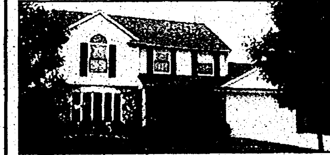
MANY UPGRADES in this 4 bedroom colonial on an extra deep lot. Hardwood foyer, neutral carpet, oak banister, full basement under family room. $240,000 (47TUR) 313-455-5600
