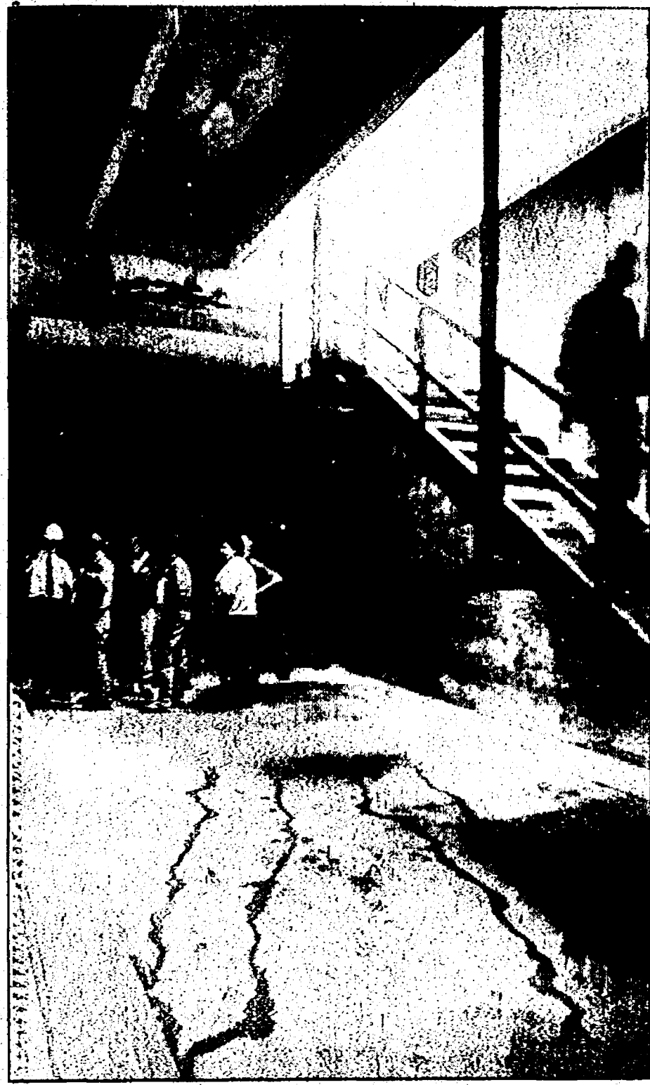
Down under: Chuck Lemont, resident engineer for Wade-Trim Associates Inc., leads guests around one of the water holding tanks at the CSO Basin in Inkster.
