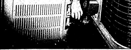
Leak potential: George Klempert, owner of Family Mechanical, Heating, Cooling & Electrical in Garden City and Madison Heights, points out where freon gas is most likely to leak, over time, at the compressor connection.
