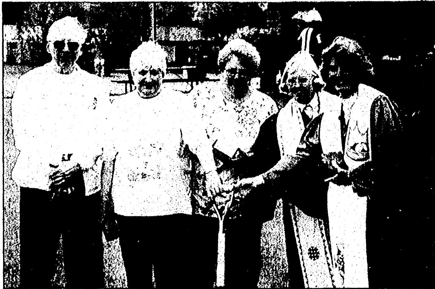
Making room: It was a banner day for members of St. Timothy Presbyterian Church when Reg Aumann (from left), Eleanor Price, Marge Riker, Rev. Dr. Anna Marie Austin and the Rev. Dr. Janet Noble broke ground for a 3,500-square foot addition to the Livonia church. The new addition will house a fellowship hall, kitchen, additional offices and restrooms. Construction will start in August with completion scheduled for August 1998.
