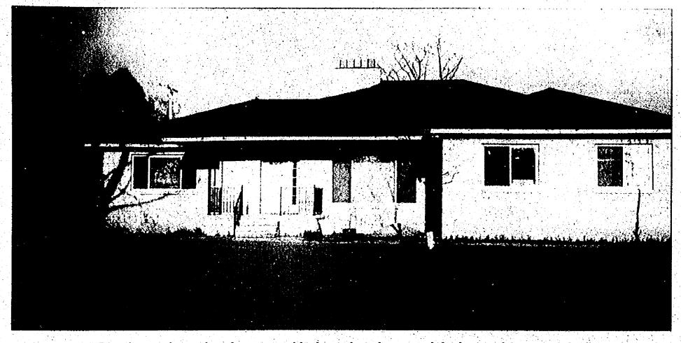
Housing twist: This house, framed with concrete blocks rather than wood, looks just like a stick-built construc-
