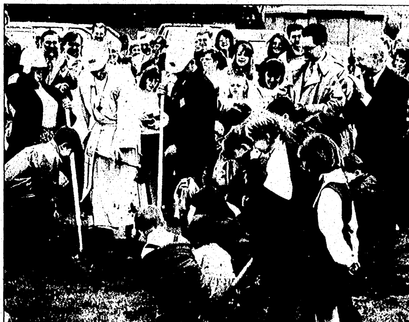
Breaking ground: Members of Holy Trinity Lutheran Church in Livonia gathered on May 5 to break ground for a new addition. Members' children helped pastors Denis Bux and Robert Seltz sink shovels into the ground for the $1.6 million addition which will include classrooms, nursery rooms, a large Fellowship Hall, administrative offices and a music rehearsal room. Plans call for the addition to be completed early next year.
