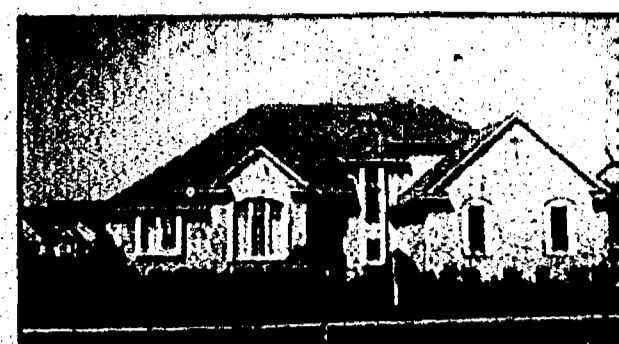
DESIGNED WITH DISTINCTION! 3 bedroom colonial with a 1st floor master bedroom and bath. Completely landscaped with paver patio, deck & sprinklers. Call today! $249,900 (50CHA) 524-1600
