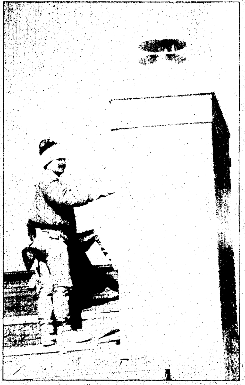
Going up: Some builders here report shortages in the construction trades, especially roughing-in carpenters. The bottom line for buyers could be higher prices.
