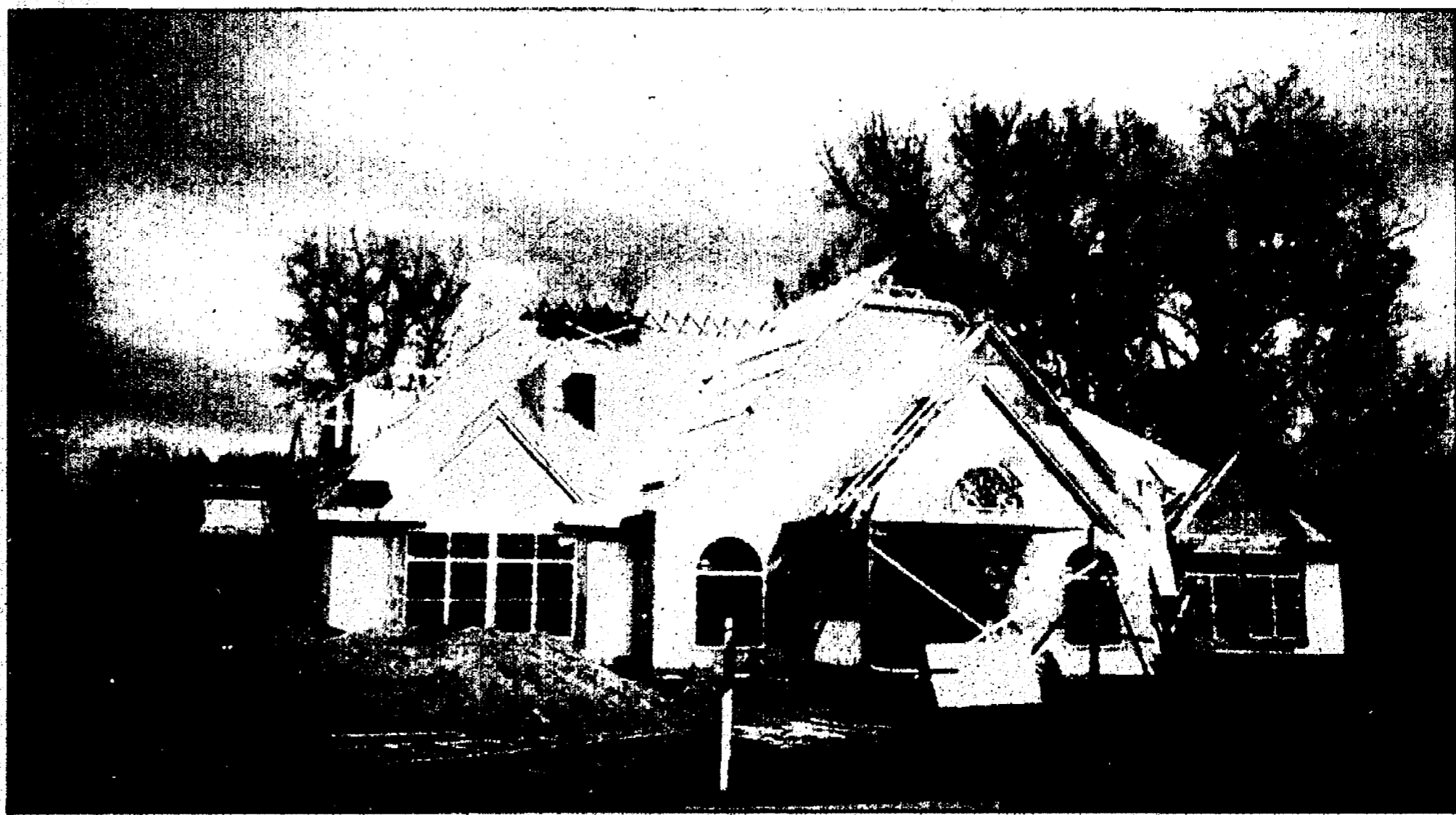
New amenity: Clubhouses, like this one under construction at Village Park of Beverly Hills, can add a new luster to older apartment complexes.
