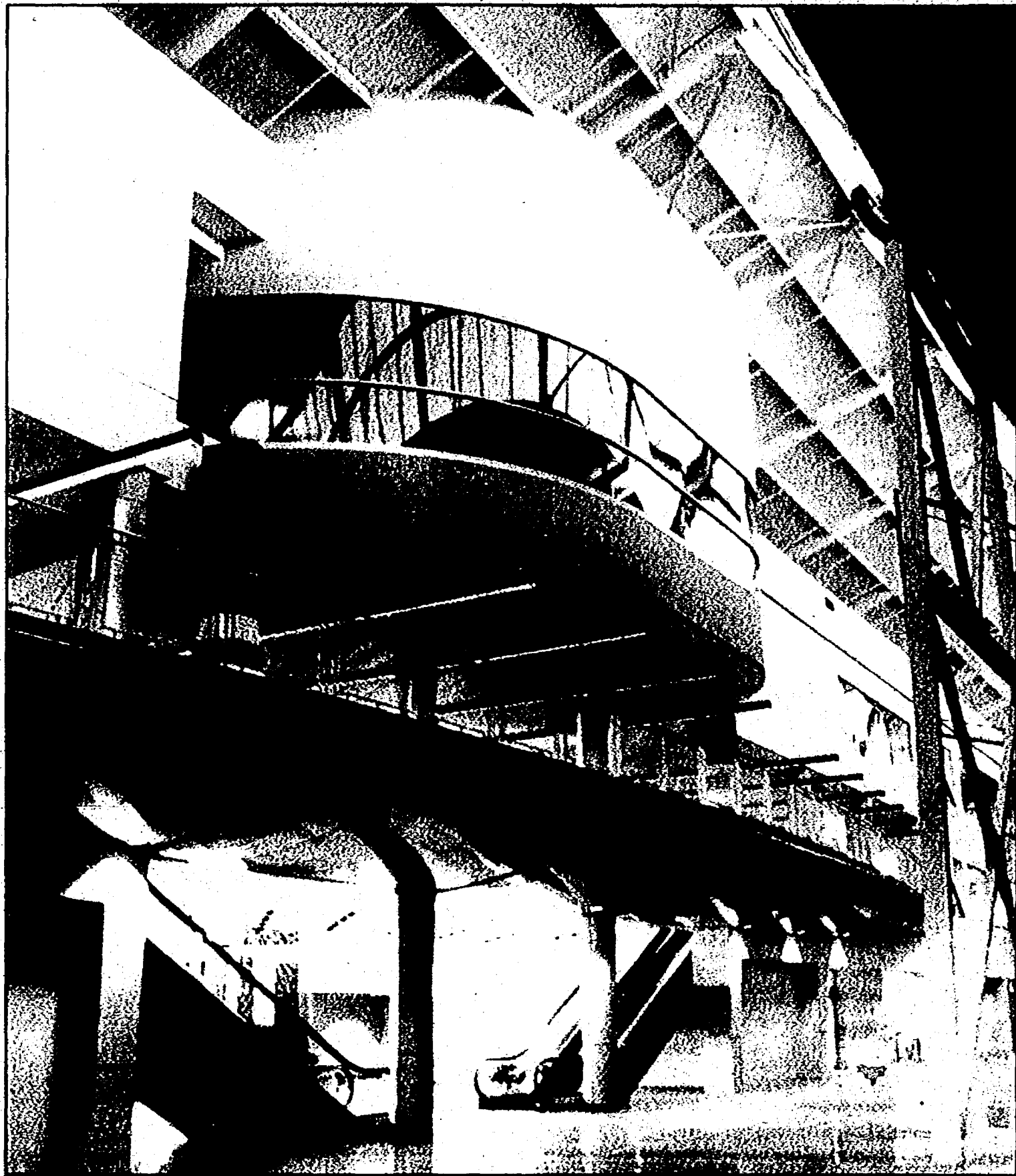
DeMattia's work: R.A. DeMattia Co. of Plymouth was the general contractor for the Focus: Hope Center for Advanced Technologies in Detroit.
