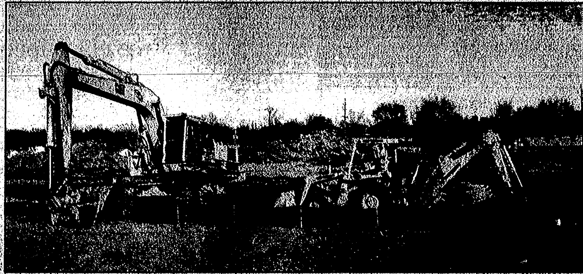
Work starts. Construction equipment and piles of dirt are visible signs that construction is under way for the new Kroger supermarket on the north side of Ford Road at Central City Parkway, opposite city hall. The work began in December after city council approval in September. The new store will replace two existing stores within a mile of the new structure. Leases for the two existing stores will expire this year. When the new store opens this summer, it will have 60,000 square feet of space, or nearly three times the size of the existing stores with other retail businesses to be part of the 12-acre site.
