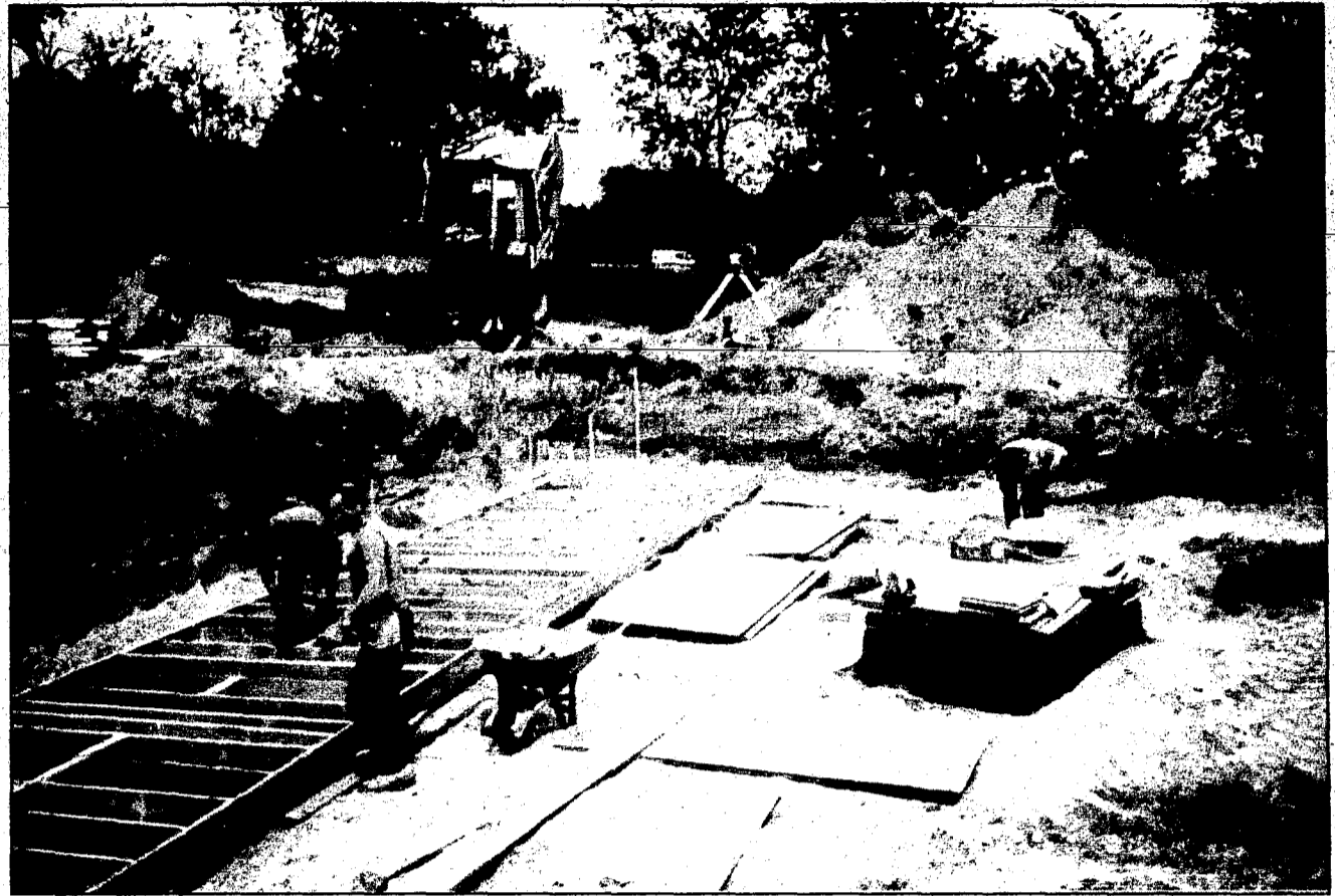
From the bottom up: Carpenters begin at the beginning by preparing the wood basement foundation.
