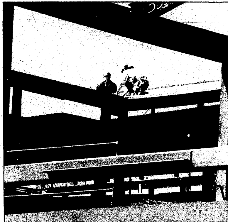
Going up: Construction workers toil on the structure of Bloom-Wood Centre set for completion in November.
