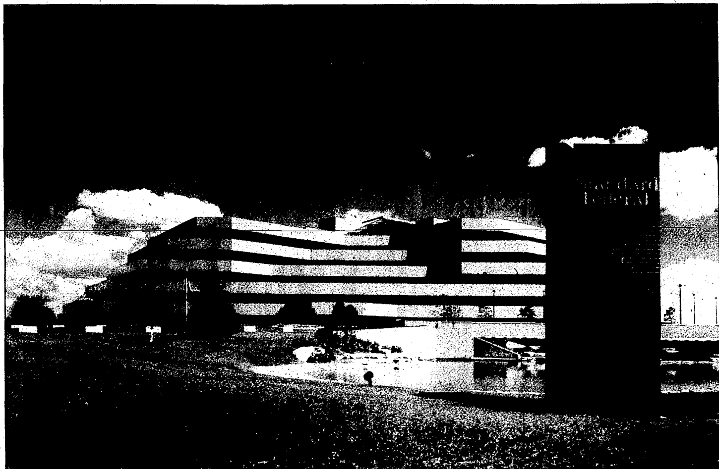
The present: The Standard Federal Financial Center in Troy was completed in 1989 and has 450,000 square feet of office space.
