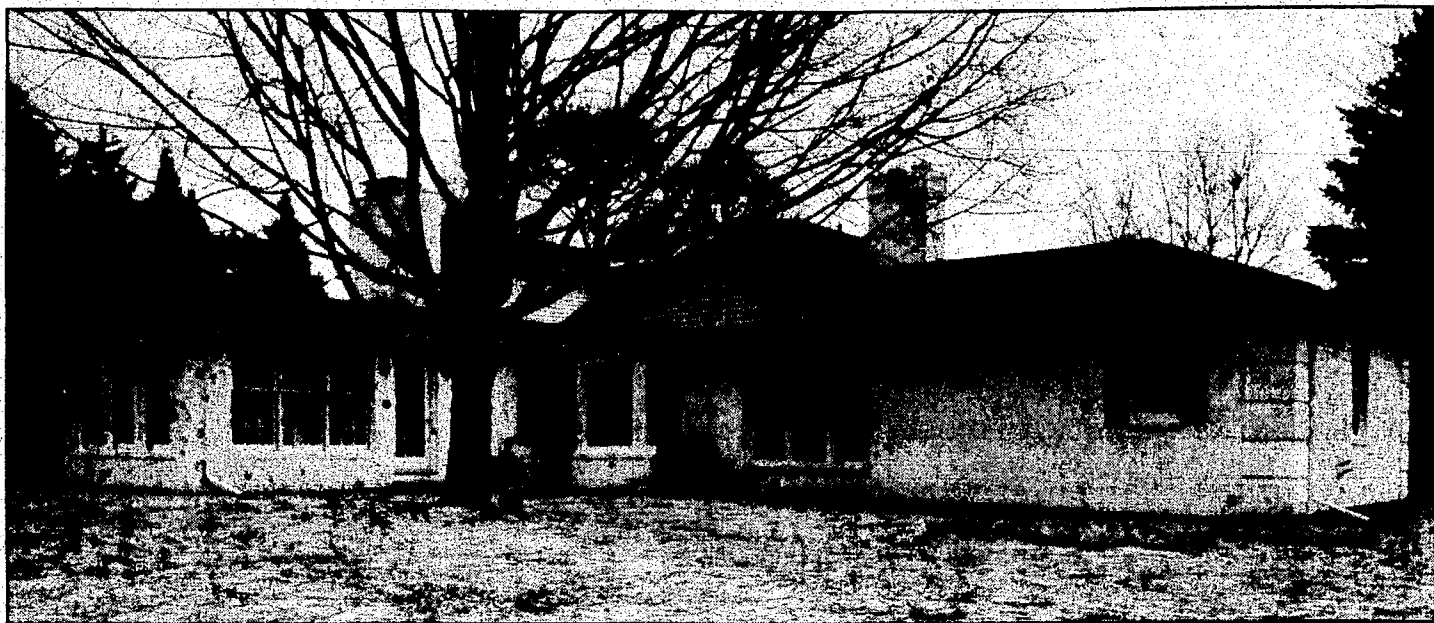
Living space boosted: This Bloomfield Village house, a two-story brick Georgian-style colonial, received an addition of 1,100 square feet to the original 3,100. The central entrance faces east (top). The additions were placed on the south and west sides of the house (bottom). A four-foot brick wall extension was placed on the south end of the second floor to expand the bedroom there. A master bedroom was added to the south end of the house, and a conservatory, with windows on three sides, was added to a family room on the west side, or back, of the house.
