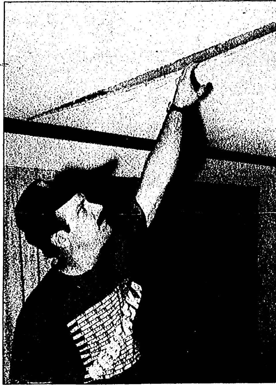
Celling problem: Randy Clark shows a crack in his mobile home's ceiling, which he claims is caused by faulty construction.
