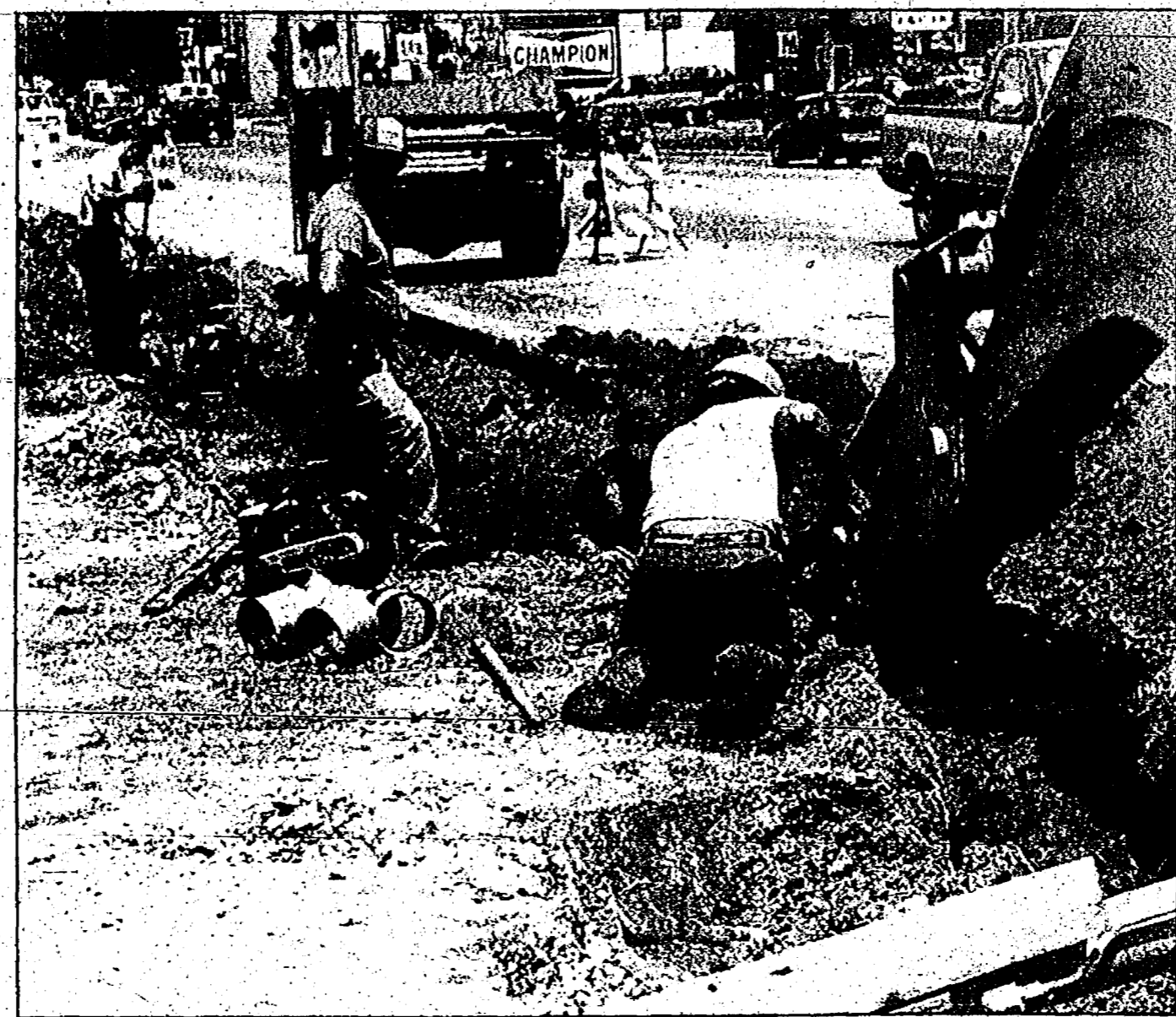
Road work: Construction crews begin the Middlebelt Road widening project by laying new drain pipes. The project, which will result in a middle turn lane, is expected to be complete by mid-September. For more about Middlebelt construction, see page 3A.
