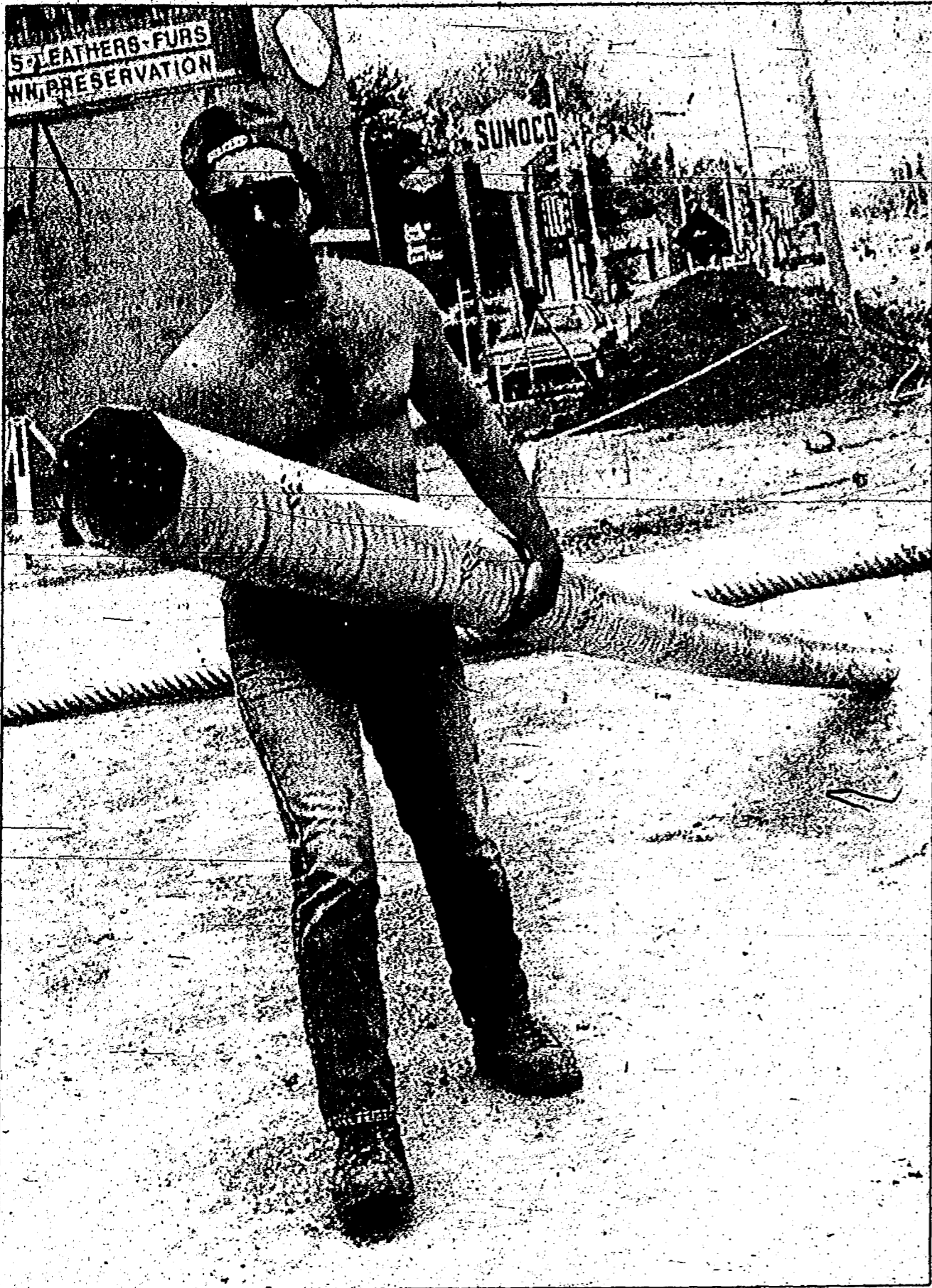
Pipe down: Construction worker Carl Glass Jr. gets ready to lay new drainage pipes. Both the edge drains and manholes have to be moved off to the side to accommodate a wider Middlebelt Road.
