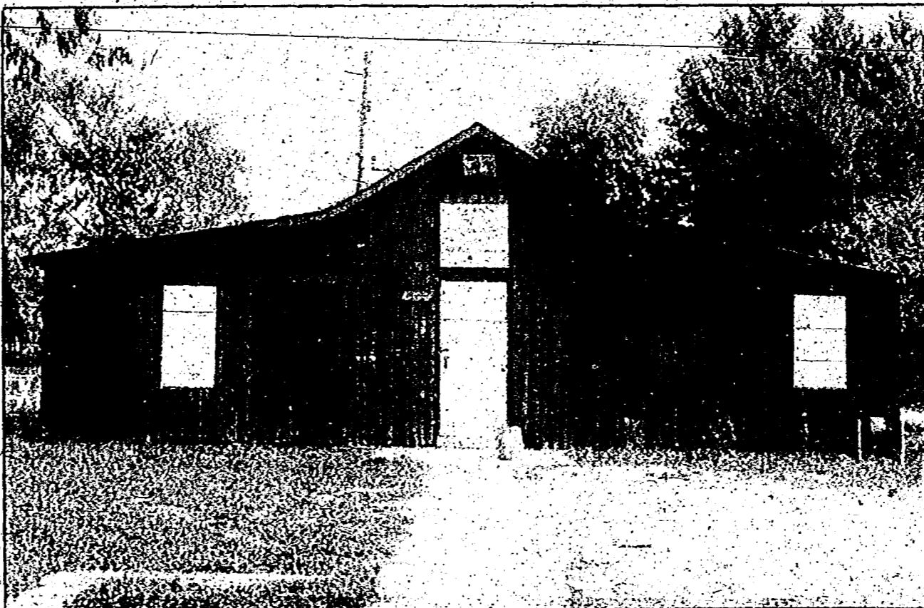
Looking back: This picture shows the Ford-Drake Scout Memorial in earlier times, before the aluminum siding job.
