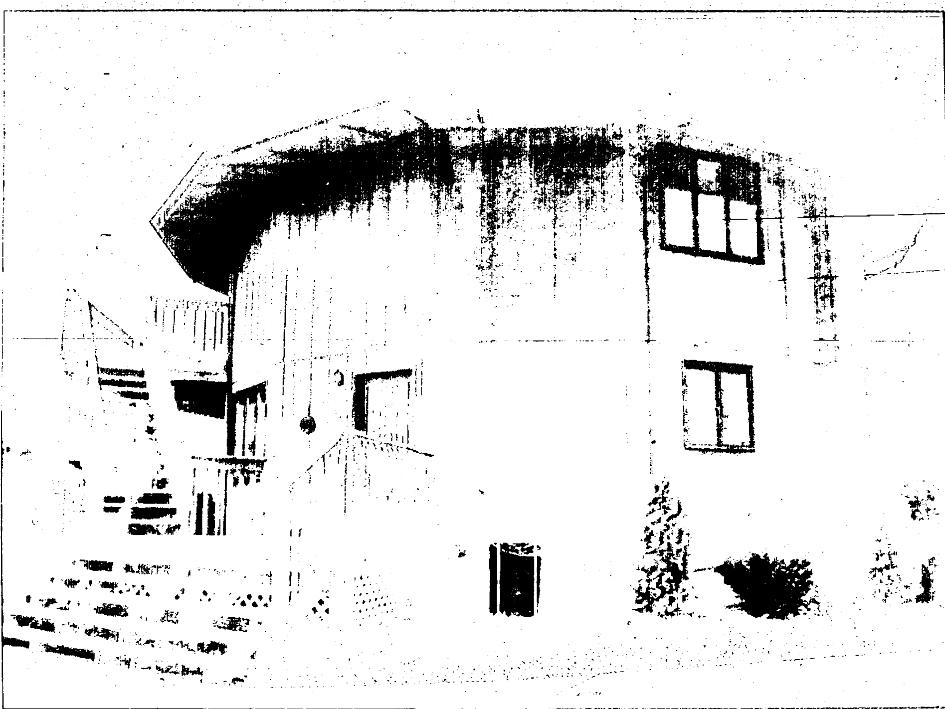
Bob and Corrine Dean's Eagles Nest House includes 14 sides and a dome-style roof topped with a cupola. The Deans built the house of Douglas Fir with cedar trim.
